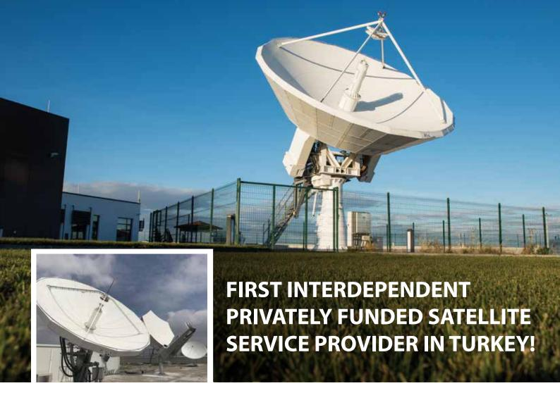
Profen Teleport Konya consists of antennas ranging from 1.8m to 11m at Ku, Ka and C band and a data centre occupying 5.000m2 of the total 25.000m2 site in Konya. The remaining area is thus available for the construction of a communications hub consisting of antennas of different sizes, data centres, equipment buildings, and containers.
